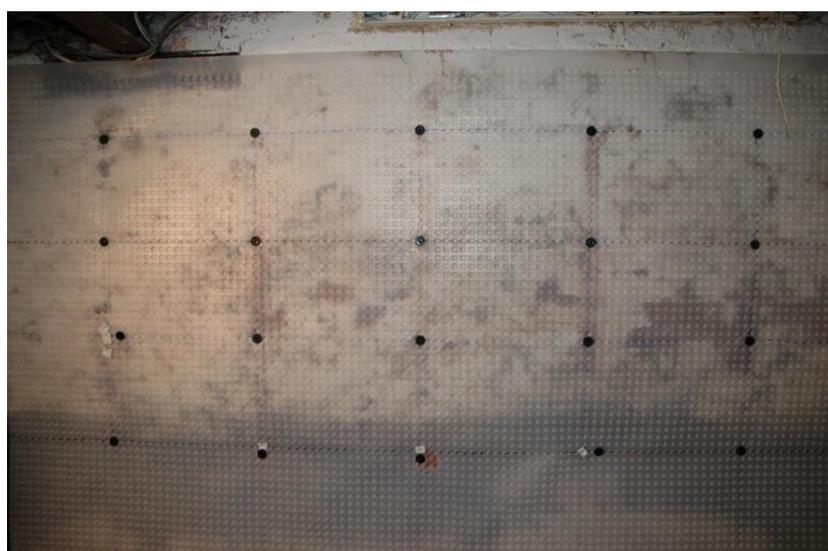
Free standing timber and metal frames and free standing block walls do not require specific fixing centres. In these cases use sufficient fixings to ensure the membrane is neat and tidy and reasonably tight to the wall, especially around corners and reveals.
