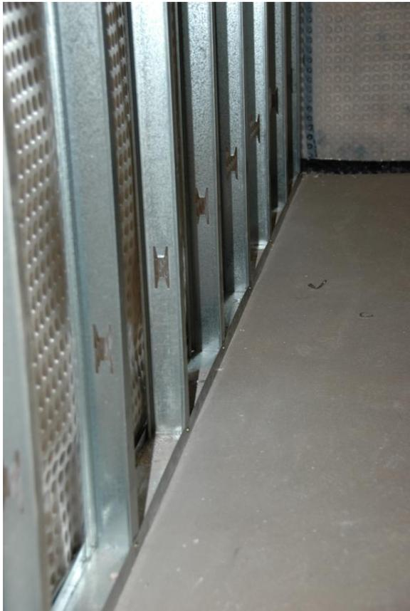
these frames in becoming more popular, the thickness of insulation required is often in excess of the thickness of the frame, and so no wall thickness is not lost when using this method.
