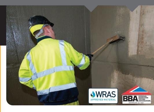
When mixed with clean water and applied correctly, Tanking Slurry forms a permanent waterproof coating to the concrete and masonry and is easily applied by brush, roller or spray.
